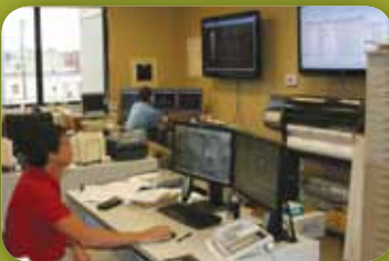
Ripley Power and Light Engineer John Perry, foreground, and Senior Engineer Chris Mooney do system planning and monitor the new load-control AdaptiVolt system through state-of-the-art SCADA equipment.
